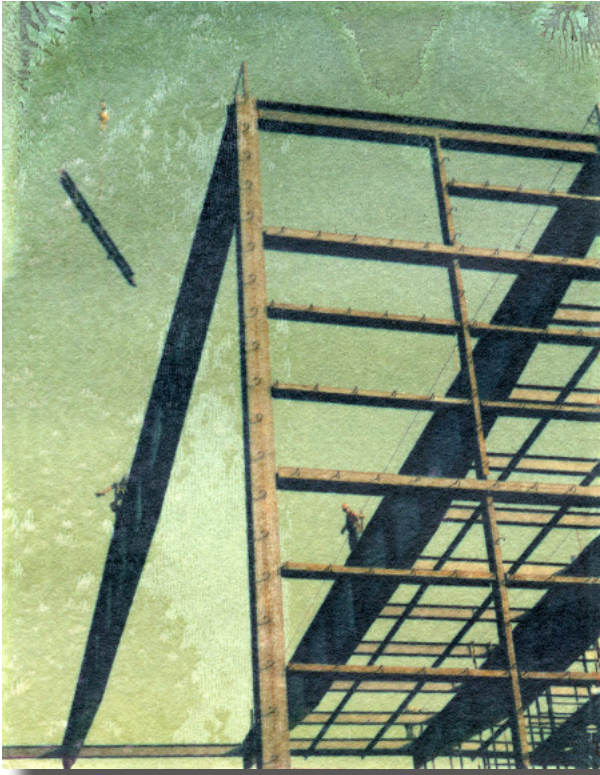
Iron Workers Series #1
