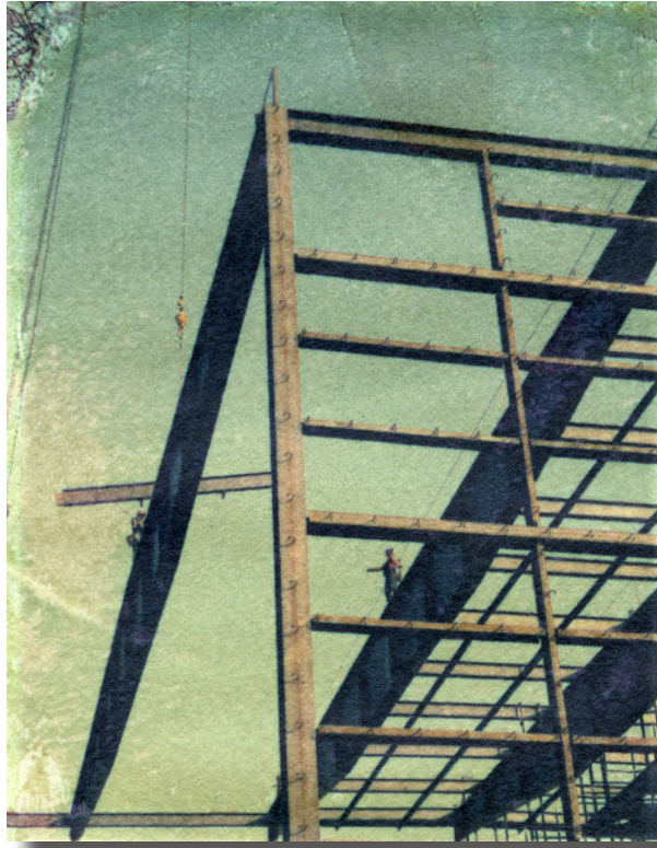
Iron Workers Series #2
